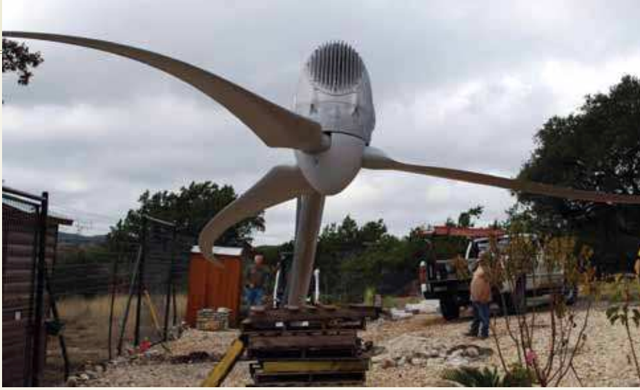
Using a winch and cable, Kevin Christiansen of RePower Energy raises a wind turbine that will generate enough energy to save the property owner about $100 to $150 each month on his utility bill.
