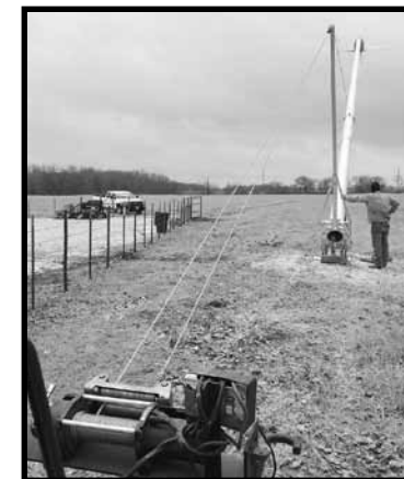
The American made Skystream 3.7 turbine is easily erected.
